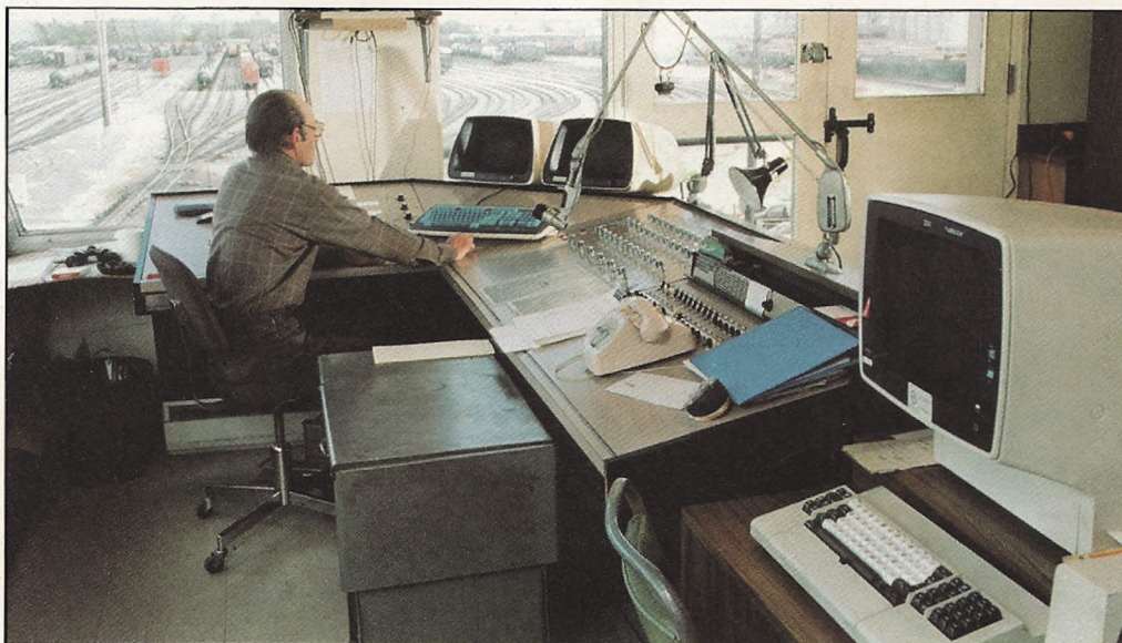
Above: From the Alyth control tower the train yard coordinator controls and monitors the entire humping operations and internal yard movements. Below: The retarder operator adds an extra measure of safety by being able to override potentially undesirable humping conditions.
