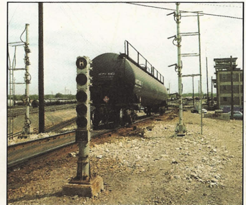
The Alyth process control system automatically weighs and humps more than 1500 cars per day to 48 different classification tracks.
