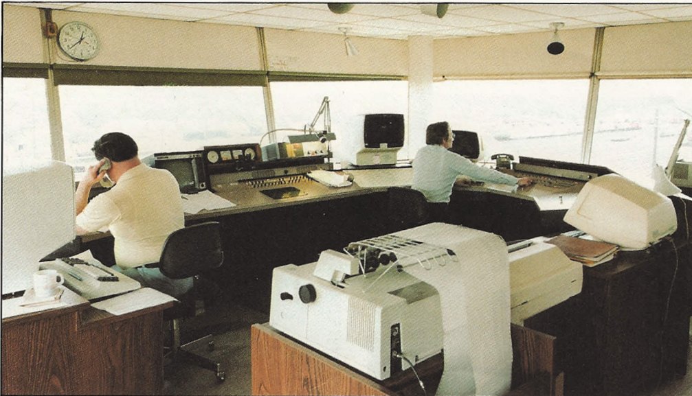
Above: From the Alyth control tower the train yard coordinator controls and monitors the entire humping operations and internal yard movements. Below: The retarder operator adds an extra measure of safety by being able to override potentially undesirable humping conditions.
