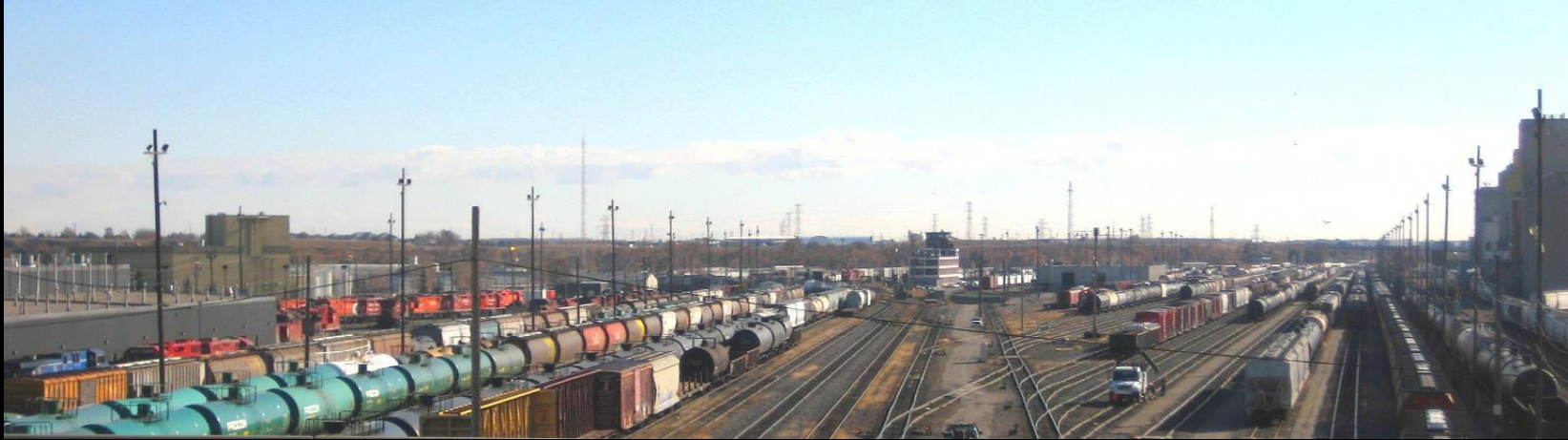
The eastern part of Alyth Yard as seen from the Blackfoot Trail overpass. L to R: diesel shop & service tracks, 'N' Yard, Hump lead heads to General Yard Office/Hump Control Tower, One Spot Car Repair Shop, 'V' Yard, 'P' Yard & Main Line to left of power line.
