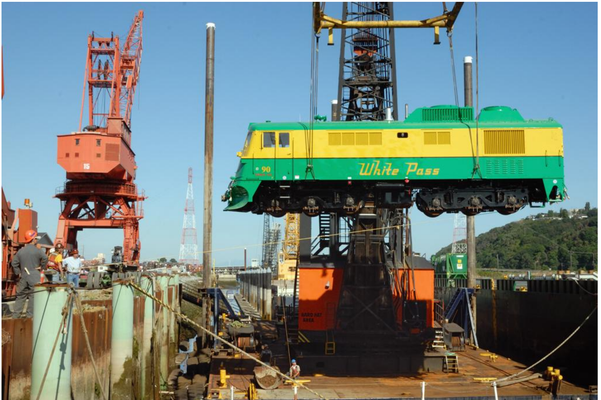
The 140 Tonne floating crane of American Construction is used to lift the second rebuilt 90 Class unit from the dock to the barge Southeast Provider. Tacoma, WA 7/21/09 Photo by Deane Motis
